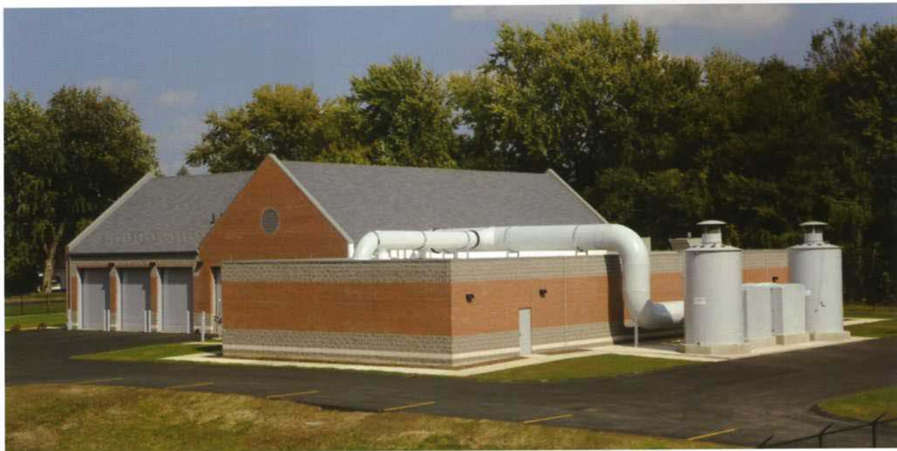
ENVIRONMENTAL IMPACT: The recently constructed $14.3 million Jones Ferry CSO Treatment Facility in Chicopee, MA, designed by Tighe & Bond, is an important milestone in the city's effort to clean up the Connecticut River.
