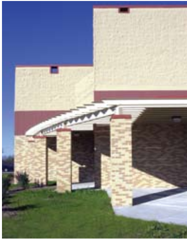
Friess Lake Elementary School, Friess Lake, WI.
