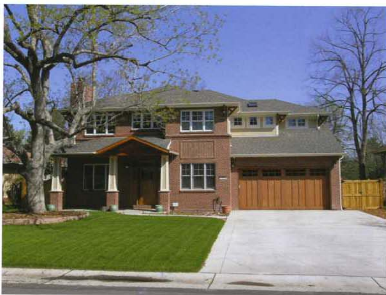
Custom home in the Crestmoor neighborhood built in the craftsman style, so that it would fit in with the homes around it. Working around the giant maple tree in the front provided a challenge in keeping the tree healthy while the house was built behind it.
